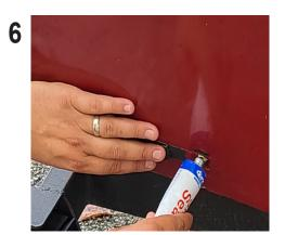
Use any marine grade silicone, adhesive or sealant and fill in the holes. Apply just enough to fill the holes. There is no need to apply any to the back of the product.
