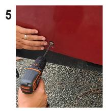
Using a 7/32" drill bit for fiberglass and a 3/16"drill bit for aluminum and wood transoms, drill out the marked holes. Put a piece of tape 3/4" up on drill bit to get the correct depth.
